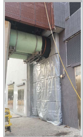
Workshop Noise Barrier
