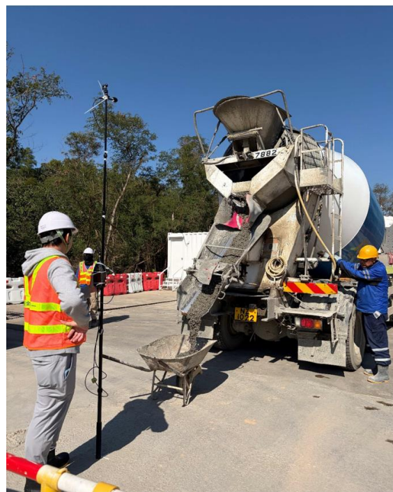
Figure 2 Photo of noise measurement (2)
