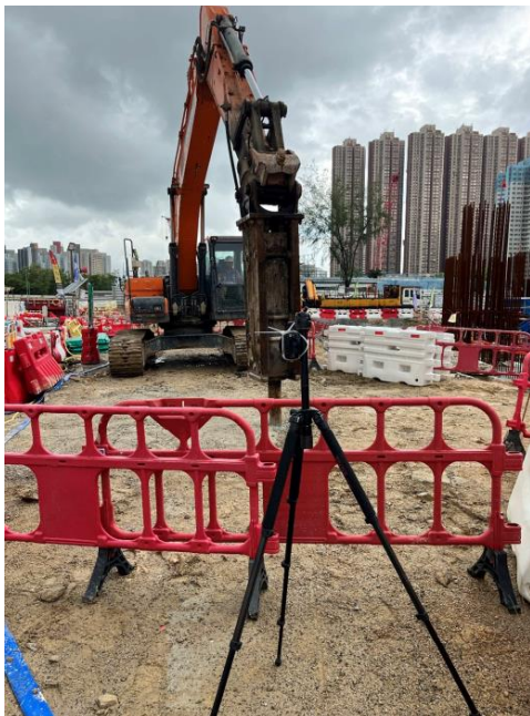
Figure 1 Photo of noise measurement (1)
