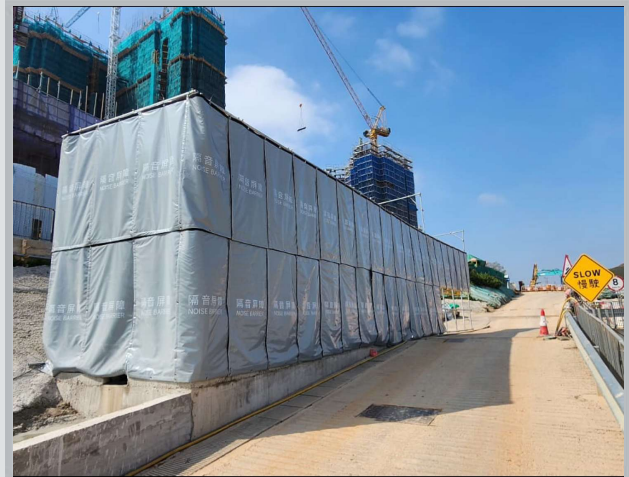
MTR Construction Site
