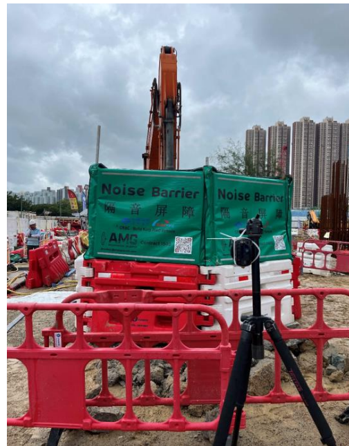
Figure 2 Photo of noise measurement (2)
