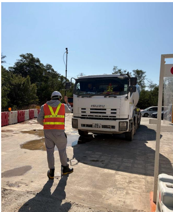
Figure 1 Photo of noise measurement (1)
